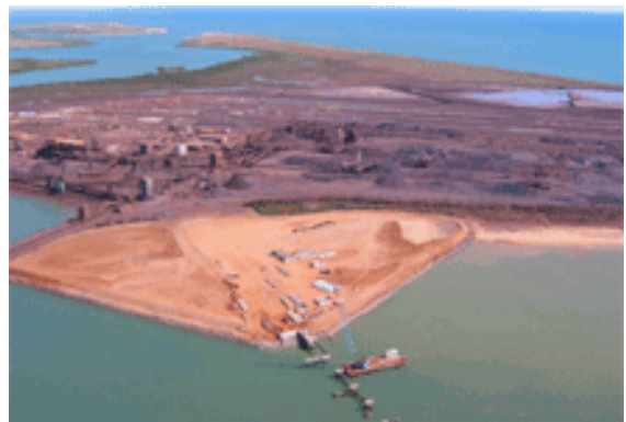
PACE) project for BHP Billiton Iron Ore
